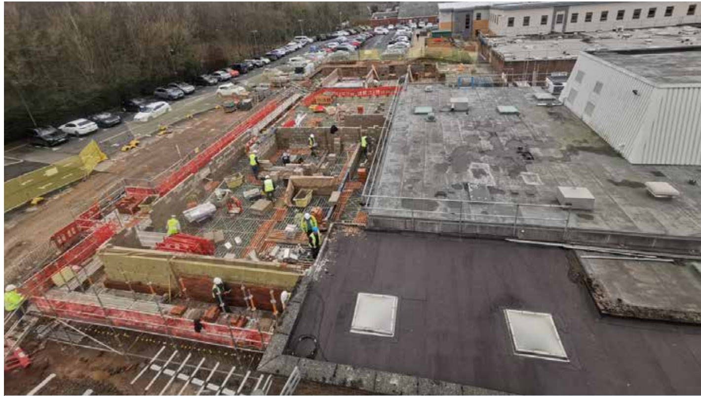
Work taking place on the new Community Diagnostic Centre, Leigh Infirmary
