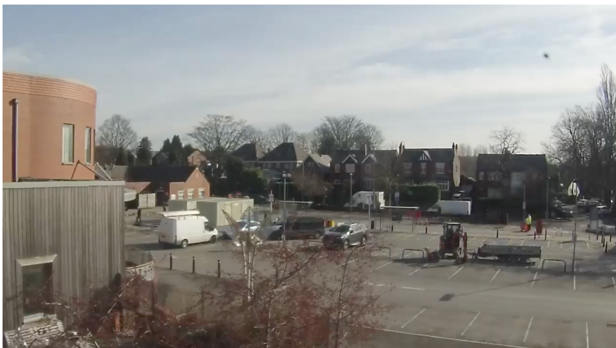
Before: The contractors beginning to arrive on site
